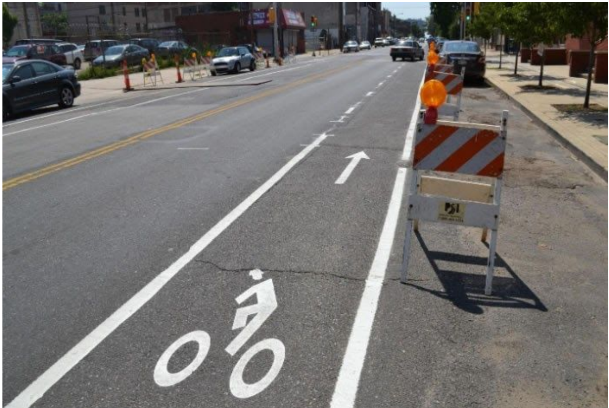
This is a dashed bike lane. As you can see the line is straight but then turns into a dashed bike lane where drivers can merge over to turn at an intersection, as long as they make sure the bike lane is clear.
